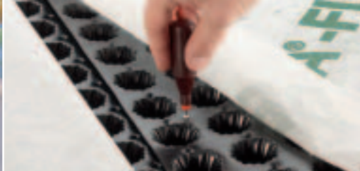
Joining sheets with DELTA®-FLORAXX connecting elements.
