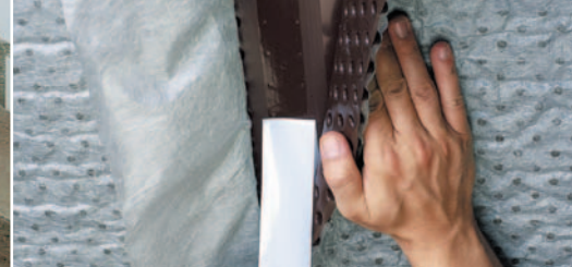
Integrated self-adhesive border for precise installation.
