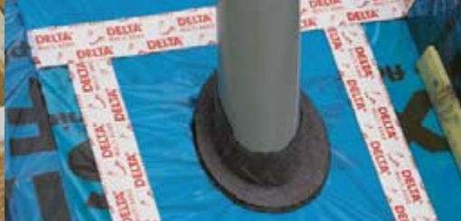
Install DELTA®-S d -FLEXX and seal against draughts.
